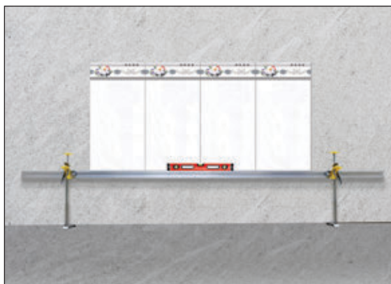
Aluminum bar supports the stone slabs during paneling process
